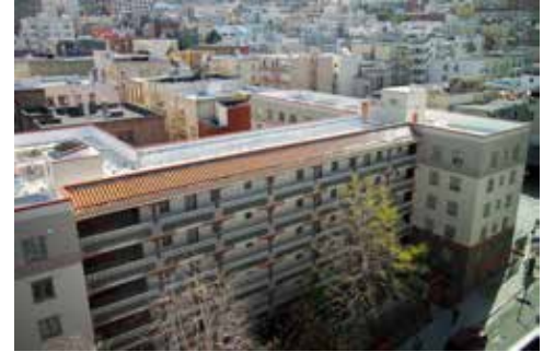
Ping Yuen, a RAD housing renovation, San Francisco, CA.
