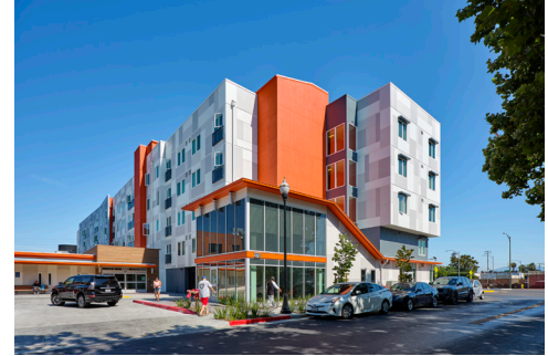
Park Avenue Senior Apartments, San Jose, CA.
