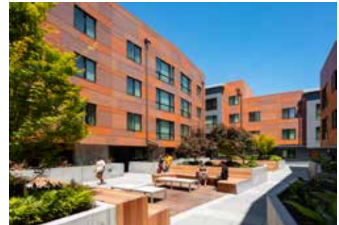
Laurel Grove Apartments, low income family housing. San Jose
