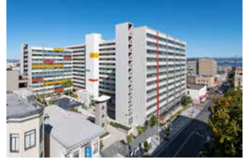
Ping Yuen North, a RAD housing renovation. San Francisco, CA.
